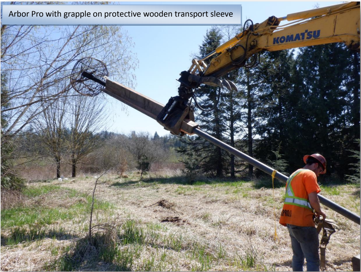
Moving the structure to the buried base
